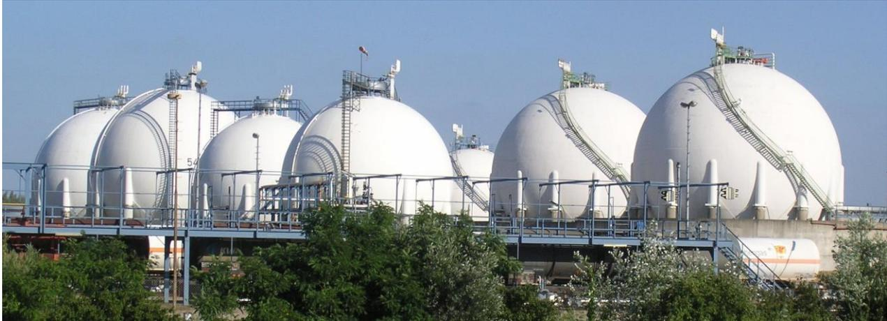
A chemical plant is realized by a continuous mass flow from the input storage to the output storage, in case of gases or liquids, the storage area is a tank farm. To increase the mass of gases, they are either compressed or liquefied. Basically there are **three different types** of storage tanks: Pressure Tanks, Cryogenic Tanks, and Atmospheric Tanks.
